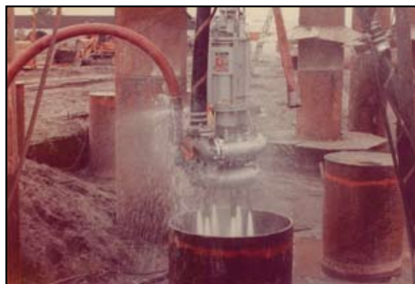
Model : DP 20 with Water Jets Application : For pumping Sand and Clay for Bridge Support Caissons Customer : USA
